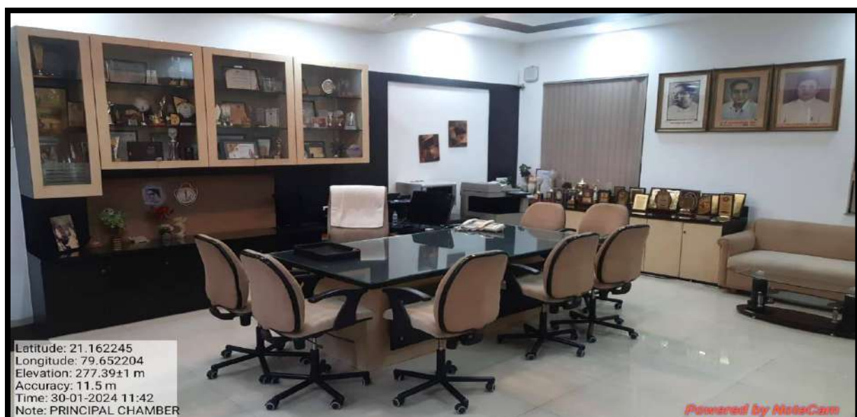
PRINCIPAL'S OFFICE WIFI ROUTER - 27
