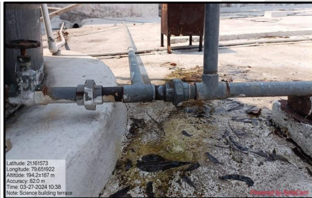
Leakages found in the Taps
