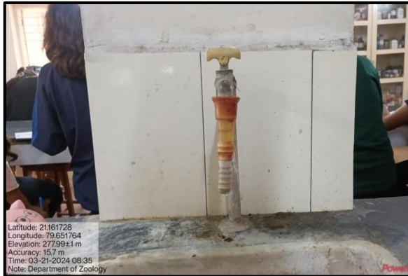
Leakages found in the Taps
